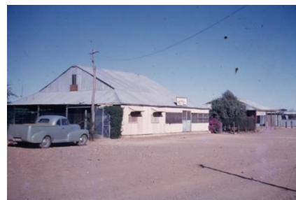
THE JUNCTION HOTEL 1960. JIM GAYTON COLLECTION
