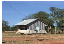
Lot 9 Fred Taylor's House (1950s)
